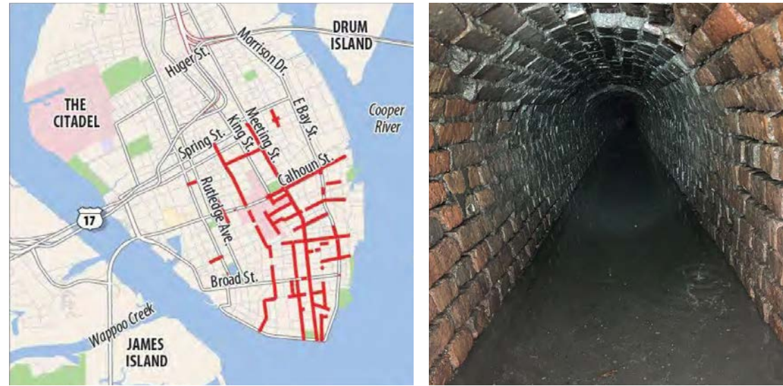
NETWORK OF CHARLESTON'S BRICK ARCHES (Source: ESRI, City of Charleston)
