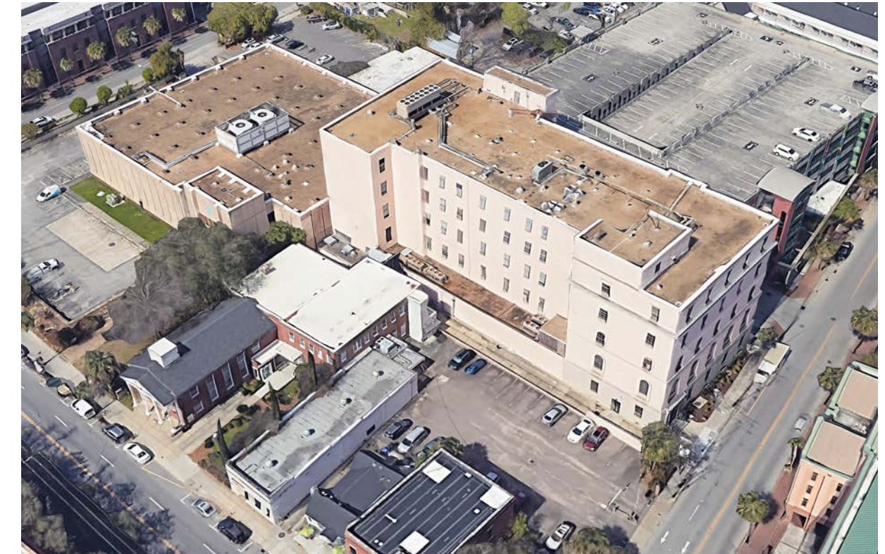
EXISTING BUILDING AERIAL VIEW
