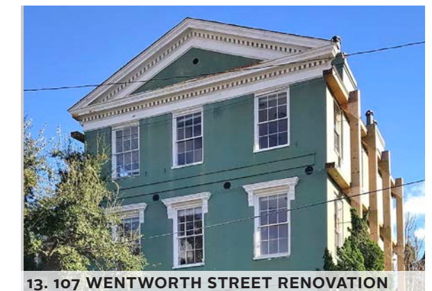
13. 107 WENTWORTH STREET RENOVATION
