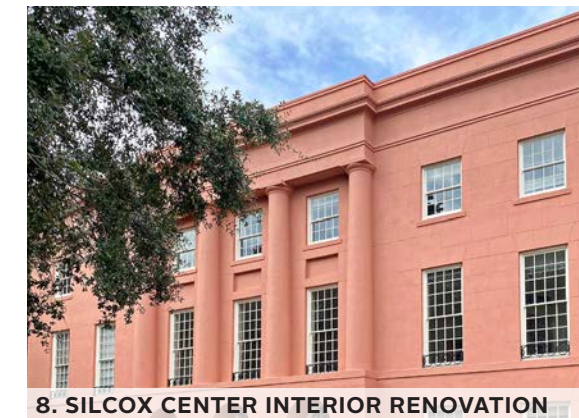
8. SILCOX CENTER INTERIOR RENOVATION
