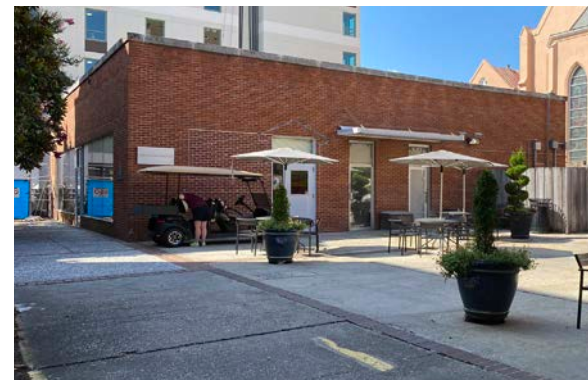
EXISTING LIGHTSEY ANNEX BUILDING
